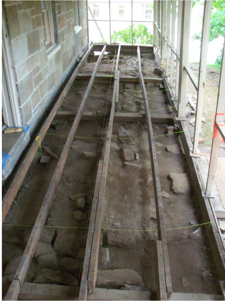
Figure 6. View of Surgeon's Quarters porch being roped off into grid units prior to excavation in 2014. (Photograph by Mark Warner)
