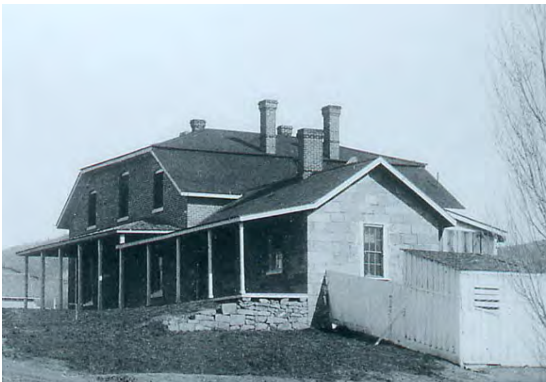
Figure 4. View of Fort Boise's Surgeon's Quarters circa 1890s—note the two-story brick addition on the left and the porch (Idaho State Historical Society Archives, Boise, Idaho).
