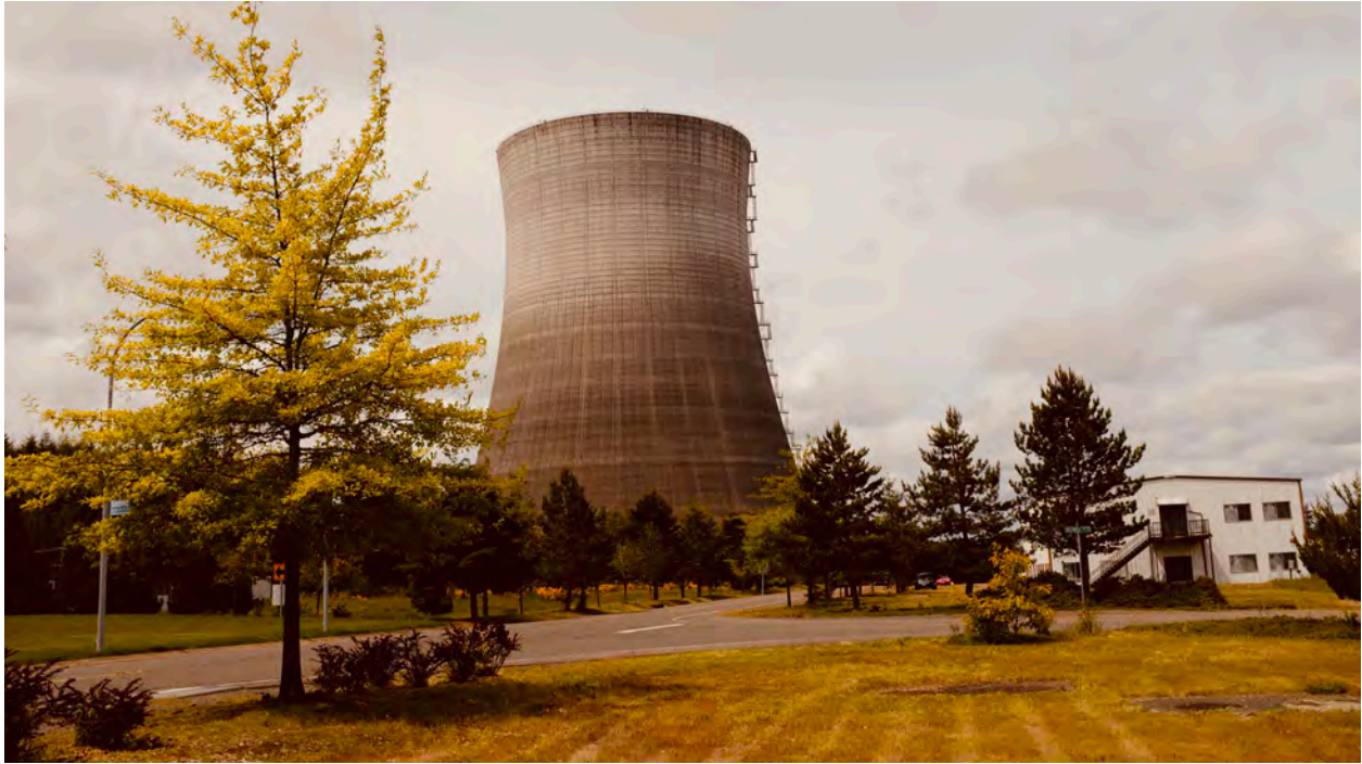
Figure 4. One of the cooling towers at the Satsop Business Park looms over the largely empty grounds of the large parcel. Photograph by Andrew Gardner, 2022.
